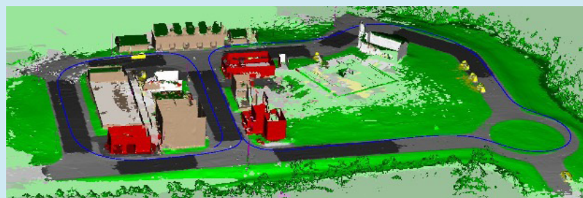
Figure 1. Computer vision techniques, such as semantic segmentation, enhance the capabilities of radiation detection measurements. A facility is segmented into distinct material classes. The trajectory of the vehicle carrying the computer vision sensors and the detectors is overlaid in blue [S85].
